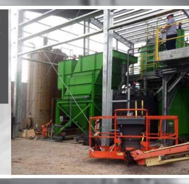
"DESIGNED SPECIFICALLY FOR INDUSTRIAL PRE-TREATMENT APPLICATIONS, ECOLOGIX CLARIFIERS SET THE STANDARD FOR HEAVY SOLIDS SEPARATION THROUGH THE SETTLING PROCESS. MAXIMAL SURFACE AREA IS THE KEY TO INCREASED SEPARATION EFFICIENCY."
